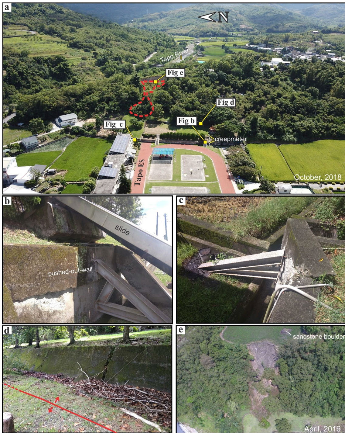
Fig. 3 Surface deformation features on the ChF-line scarp in Tapo ES area. a Oblique view of the Tapo ES area. Taken on 5 October 2018 by a camera drone. The red dashed line outlines the remains of the landslide in 2016 (see Figure e). b Tilted platform of the slide and bulging wall. c Torn apart concrete wall. d Cracked concrete wall and bulging ground. e A landslide incidence. Drone photo taken on 16 April 2016
